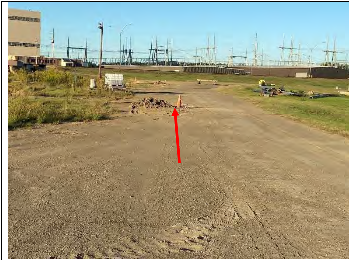
Photograph 1: View along crest, looking left. Arrow points to location of recent boring locations.
