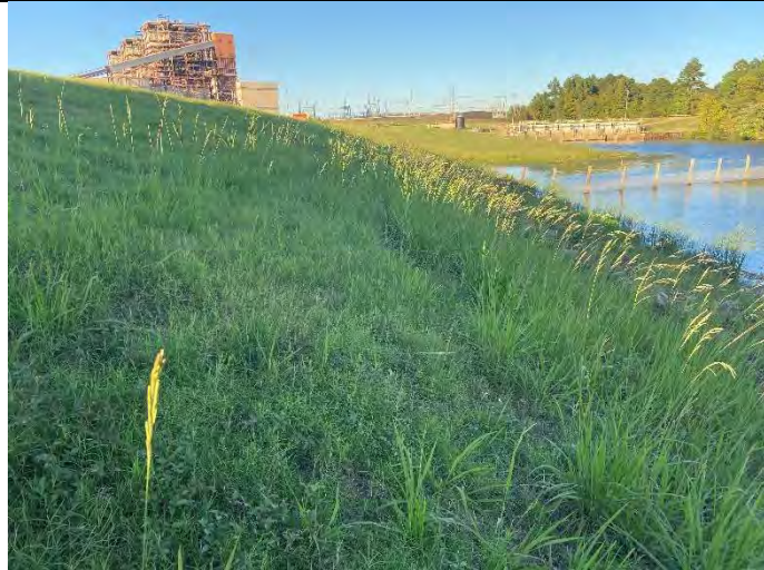
Photograph 5: Typical view of downstream slope, looking left.
