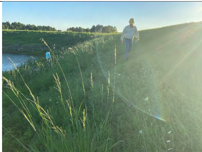
Photograph 6: Typical view of downstream slope, looking right.
