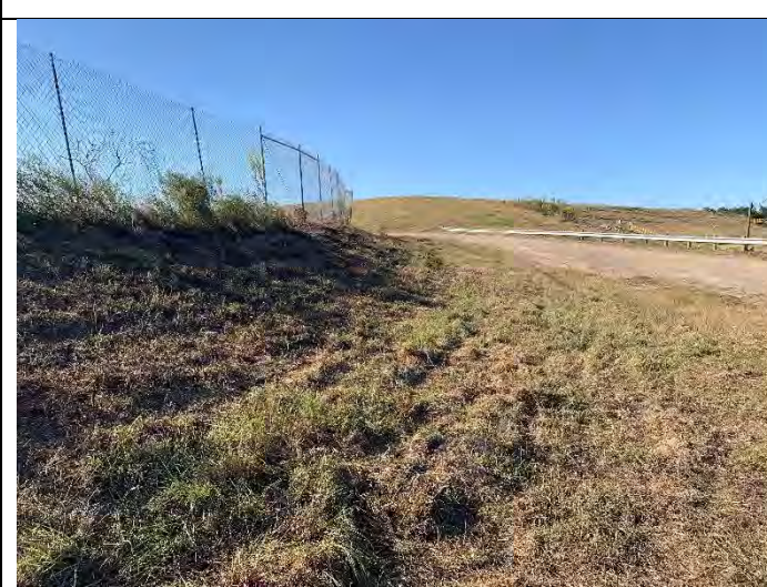
Photograph 15: Typical view of downstream slope of east embankment, looking north
