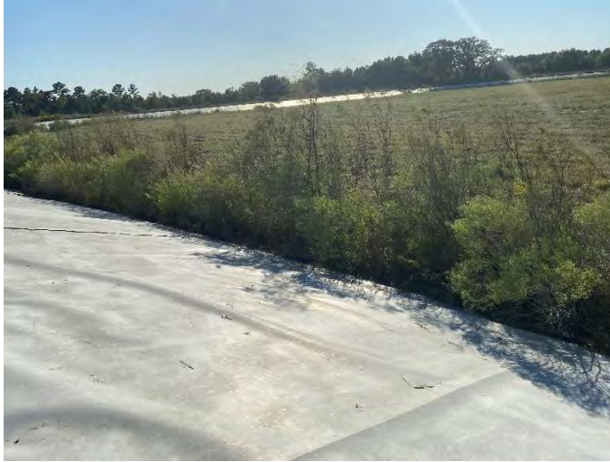
Photograph 5: Example woody vegetation growing at toe of geosynthetic liner toe-in on upstream slope.
