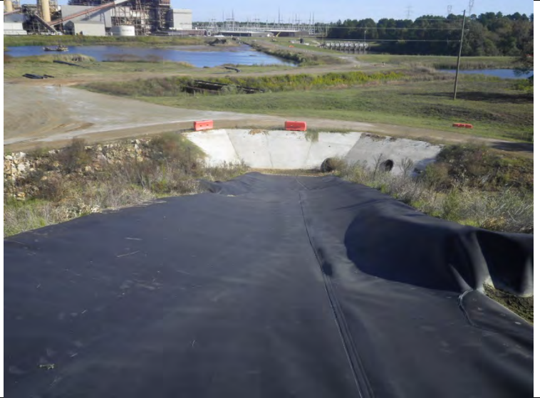
PHOTO #7 HDPE-lined letdown in northeast corner
