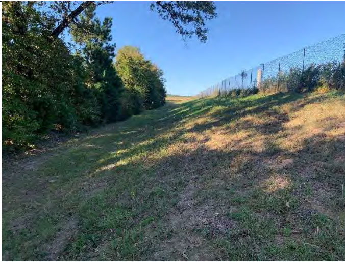
Photograph 20: Typical view of downstream slope of west embankment, looking north.
